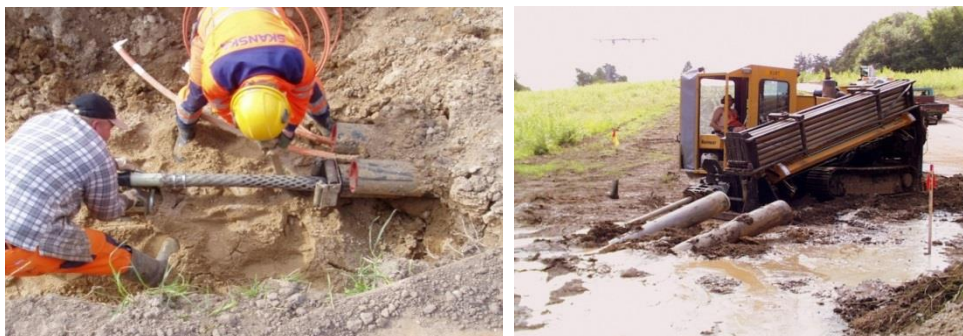
Figur 3-37 Etablering af underboring for elkabel
